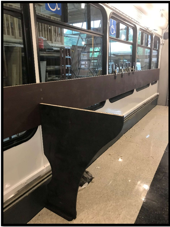
Counter supports and backsplash installed.
