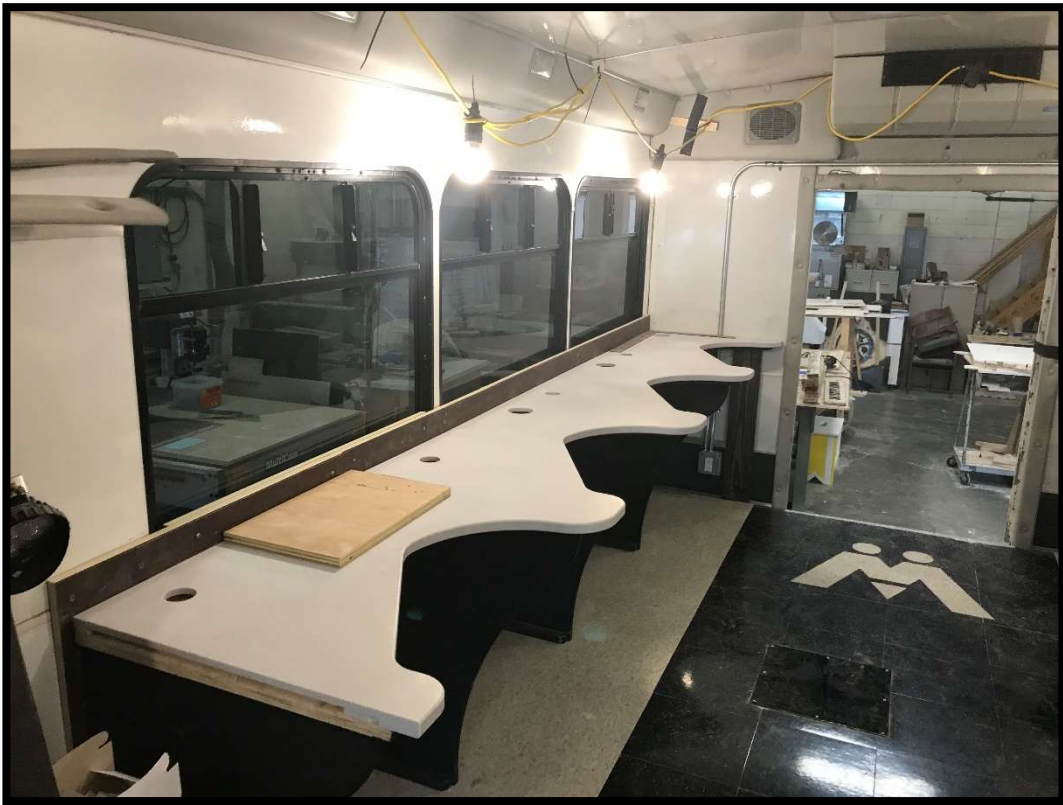
The counter supports and one-piece countertops are put into place.
